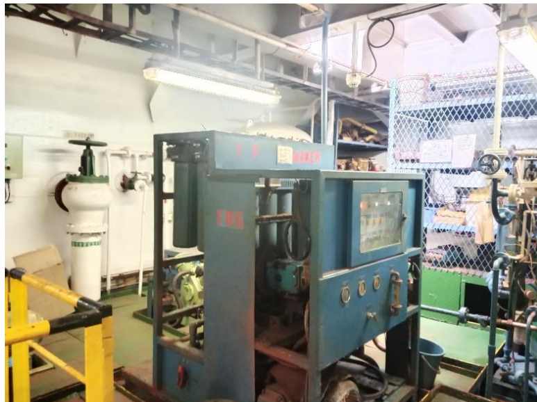
Gambar: 3. FWM STS RO SW-10T FC. Winning Sunrise Sumber: FC. Winning Sunrise
