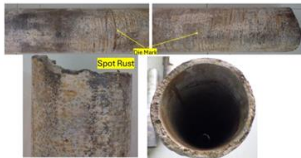
Gambar 2. Pengamatan visual sampel drill pipe B (Patahan B)
